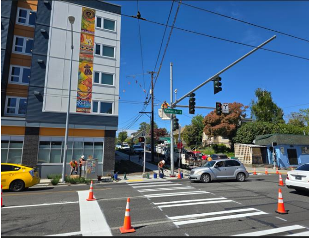
Signal major maintenance at Rainier Ave S and S Rose St.
