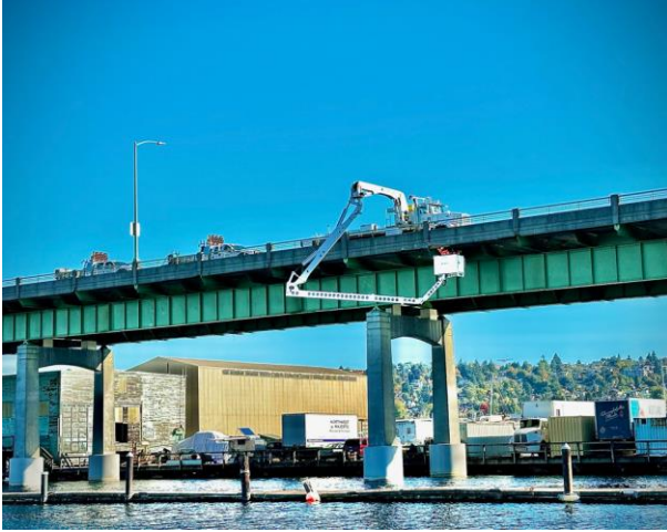
Making repairs on the Ballard Bridge.
