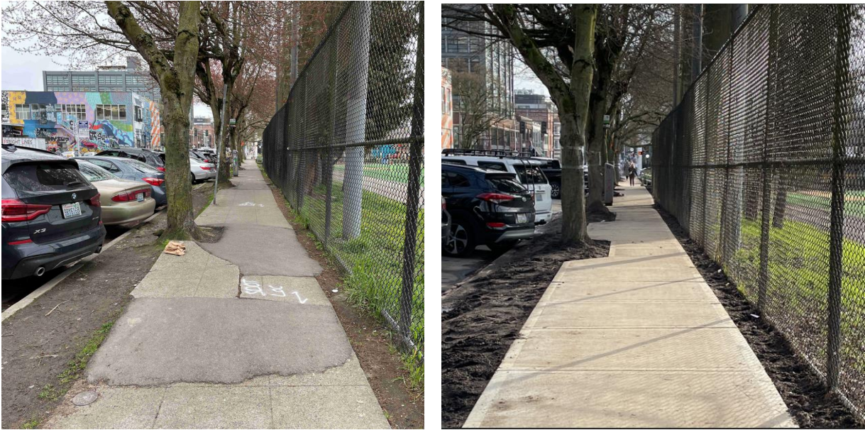
Before (left) and after (right) sidewalk repair on 11 th Ave E.
