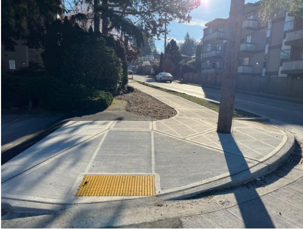
New sidewalks on NE 95 th St.
