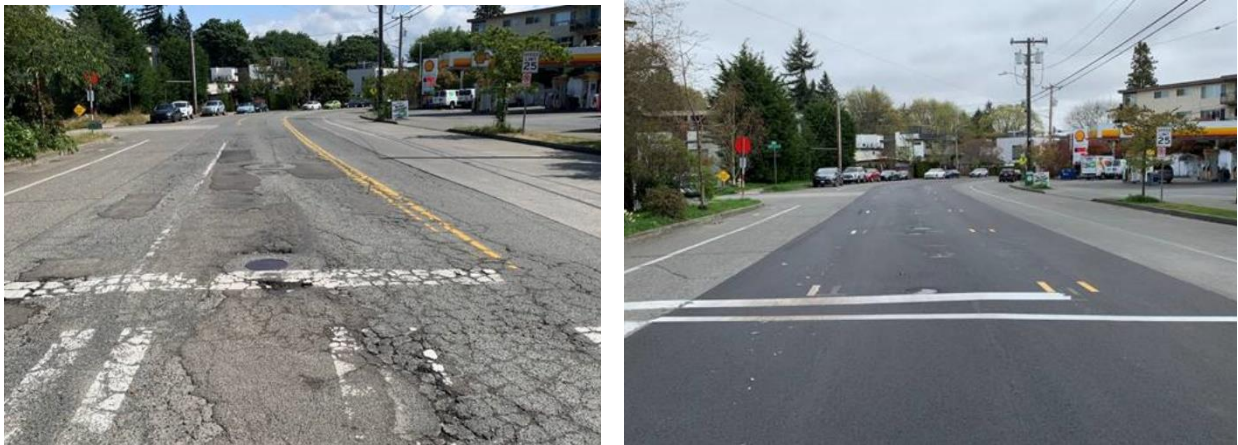
Before (left) and after (right) repaving on W Government Way.
